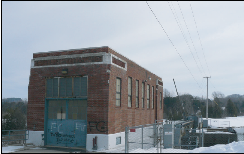
Figure 3.3.-2. Sabin Dam Power House
