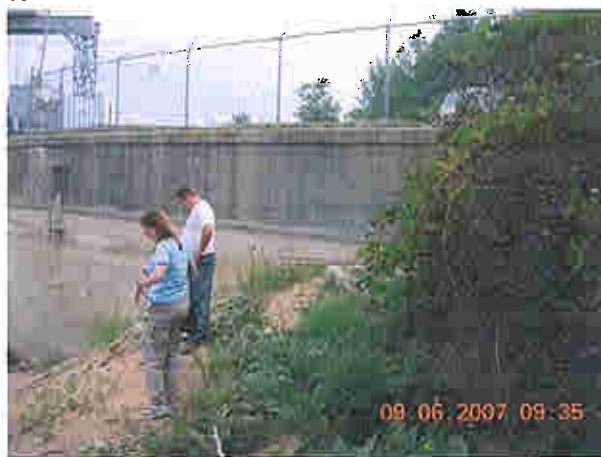
Upstream side of dam, right side
