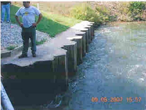
Left side downstream of powerhouse
