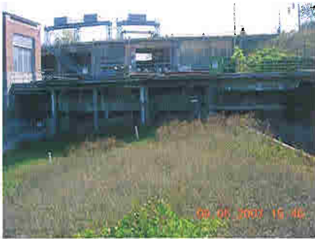
Downstream side of access deck
