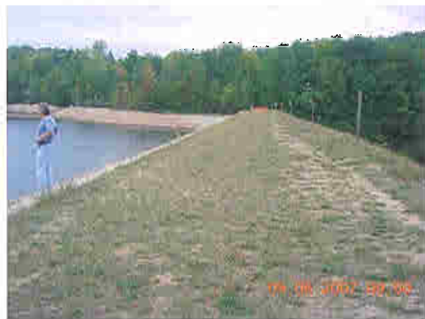
Detached earth embankment, view looking left
