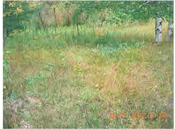
Area downstream of downstream slope of right embankment
