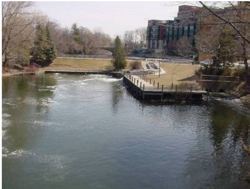
Union Street Dam, looking upstream (Not taken at time of inspection)
