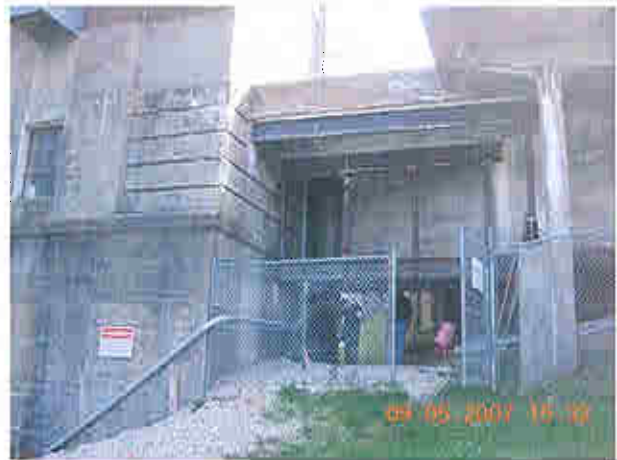
Downstream side of powerhouse and access deck
