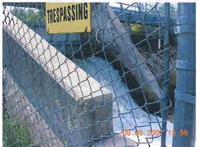
Downstream side of tainter gate spillway
