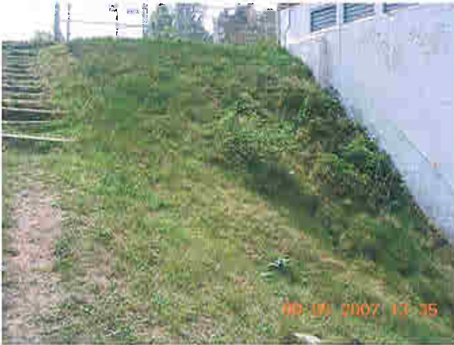
Downstream slope of intermediate embankment, near power house.
