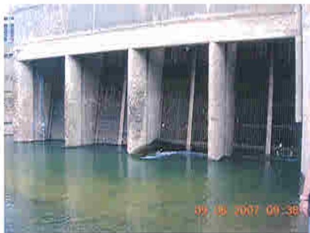
Upstream side of intakes
