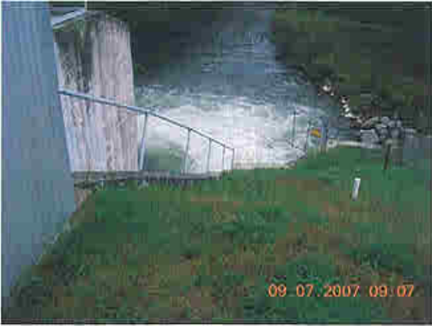
Right downstream embankment to the right of the powerhouse
