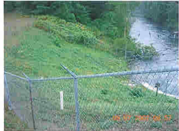
Downstream slope of left embankment near powerhouse
