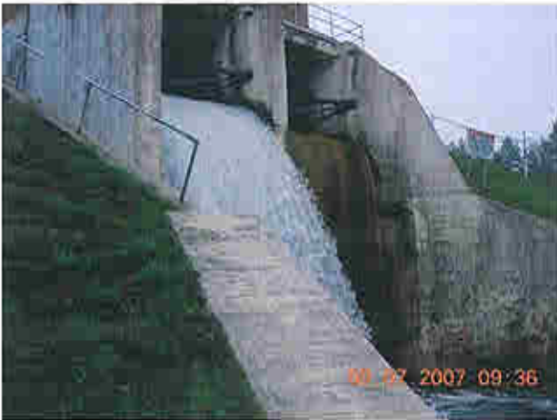
View from right downstream embankment slope
