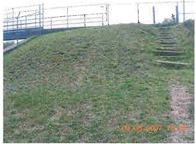
Downstream slope of intermediate embankment
