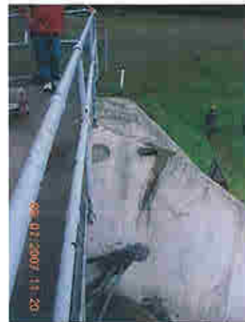
Right face of left wall of right tainter gate spillway
