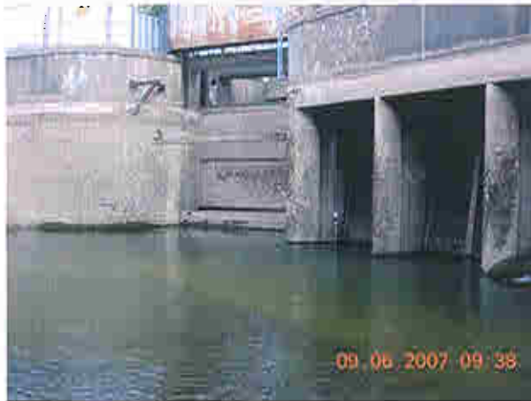
Upstream side of spillway and intakes
