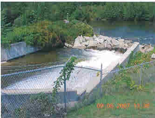
Downstream of tainter gate spillway
