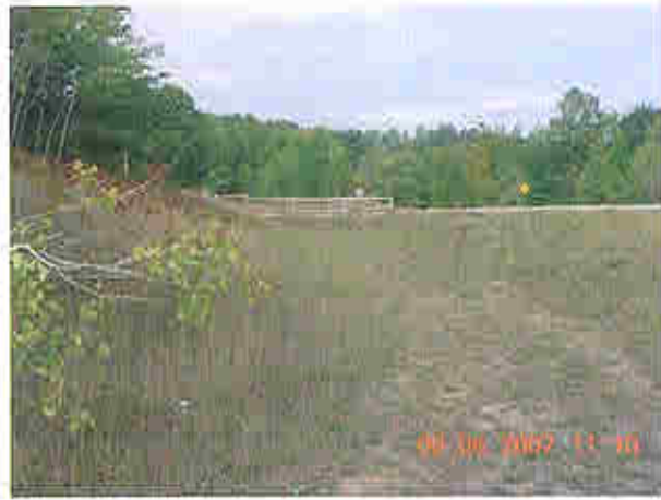
Emergency spillway, view looking left/ downstream
