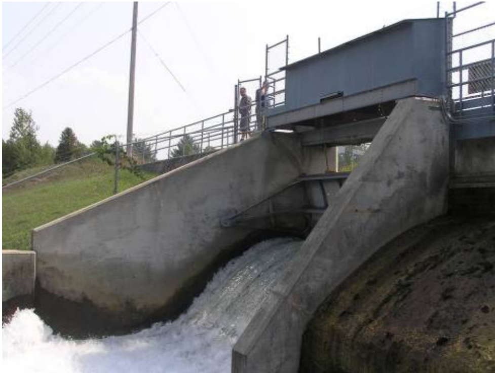
Sabin Dam Spillway
