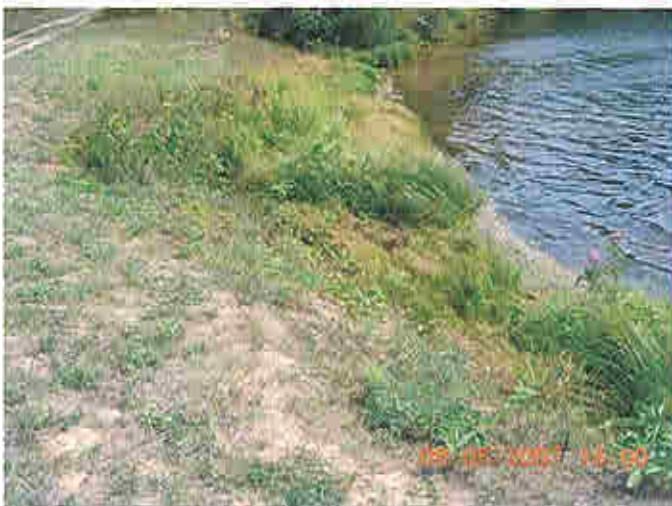
Upstream of right embankment, once eroded but since stabilized vegetated area
