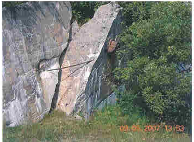
Original spillway structure, left abutment wall
