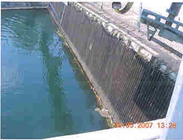
Trash racks at upstream side of powerhouse spillway.
