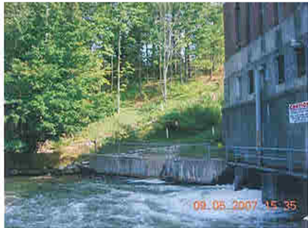
Downstream of powerhouse, view of right embankment
