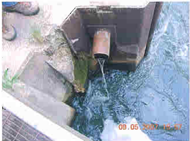
Left side downstream of powerhouse
