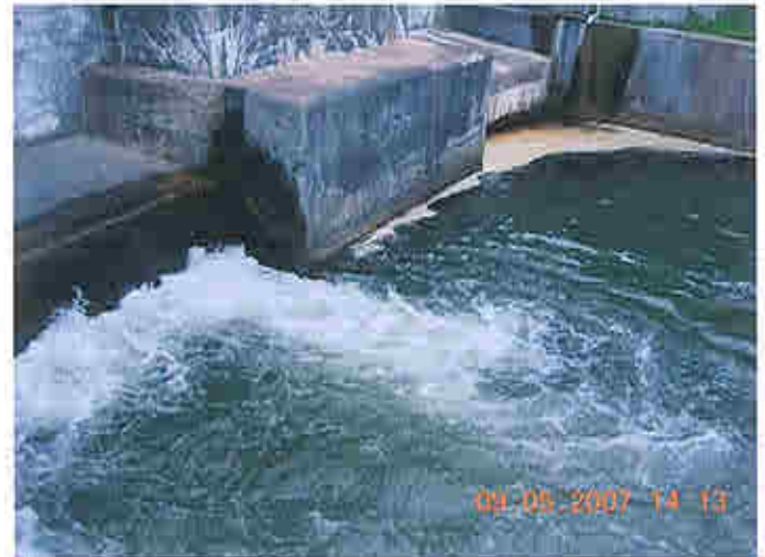
Downstream of powerhouse
