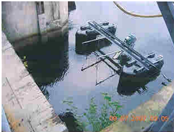
Upstream of tainter gate spillway
