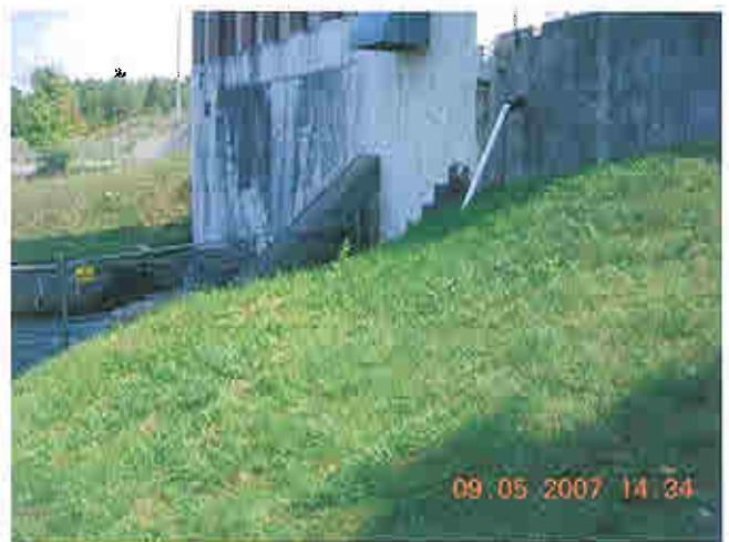
Left embankment, view looking right
