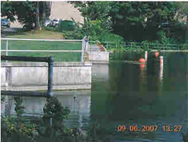
Upstream of principal spillway, view from left embankment, looking right
