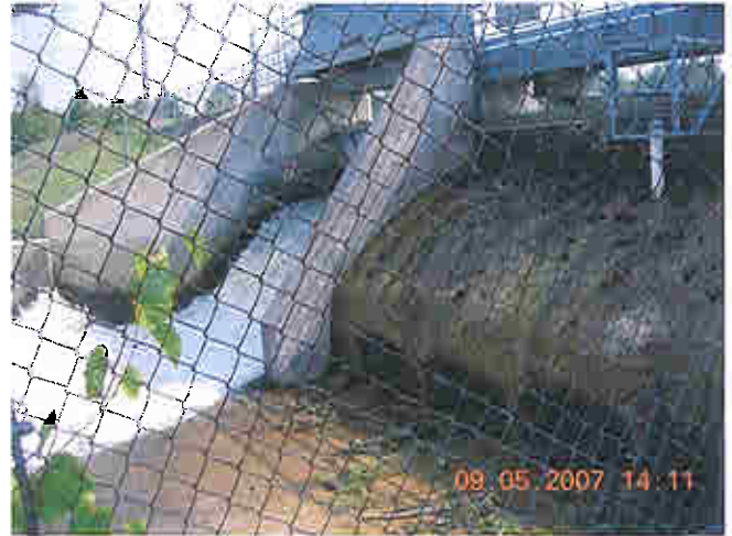
Downstream side of stop log and tainter gate spillways
