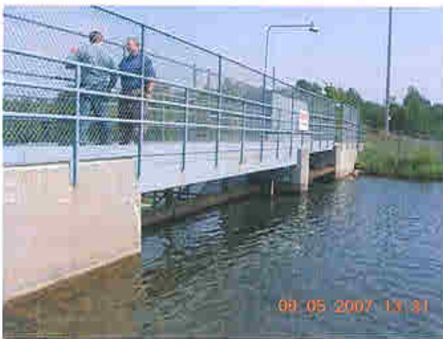
Upstream side of stop log spillway and tainter gate spillway
