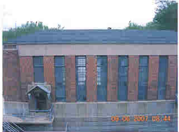
Upstream face of powerhouse
