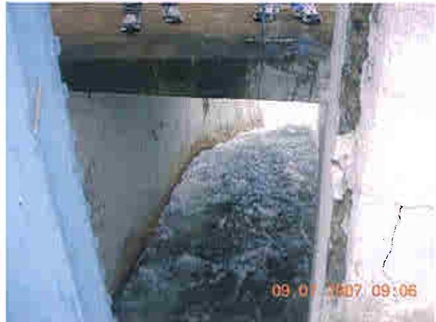
Downstream of log chute spillway, looking upstream
