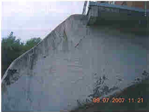
Left face of left wall of right tainter gate spillway
