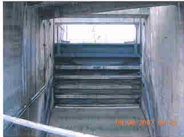
Downstream side of gate at spillway
