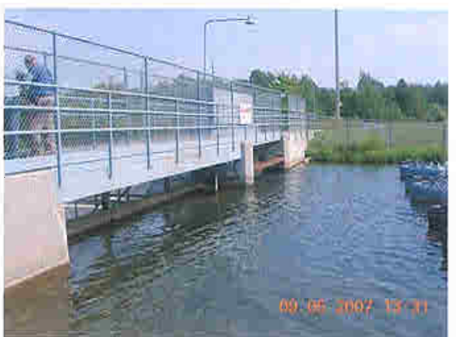
Upstream side of stop log spillway and tainter gate spillway
