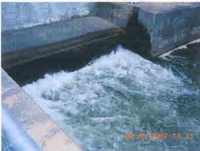
Downstream side of powerhouse
