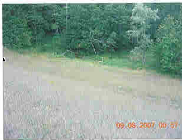
Detached earth embankment downstream slope, left end
