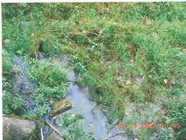
Downstream slope of right embankment
