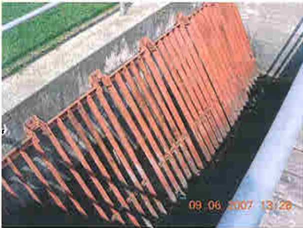
Trash rack on upstream side of inlet section of auxiliary spillway
