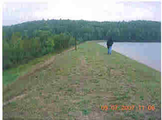
Right embankment, view looking right
