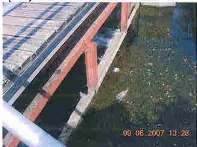
Upstream of stop log overflow section of auxiliary spillway
