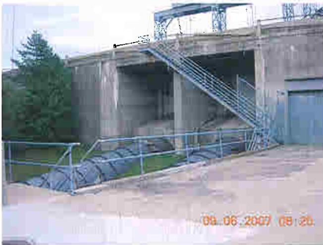
Downstream side of road, note penstocks
