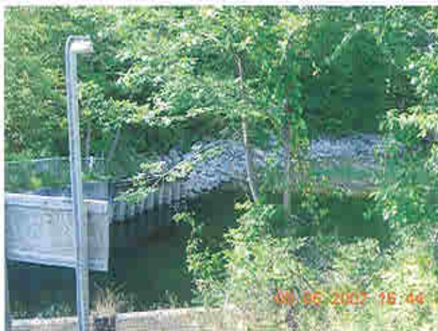
Downstream of spillway, view of left abutment
