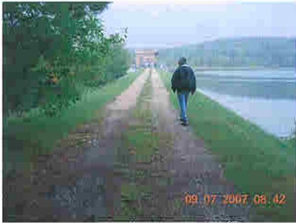
View from left end of left embankment, looking right
