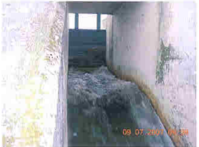
Downstream side of gate at log chute spillway
