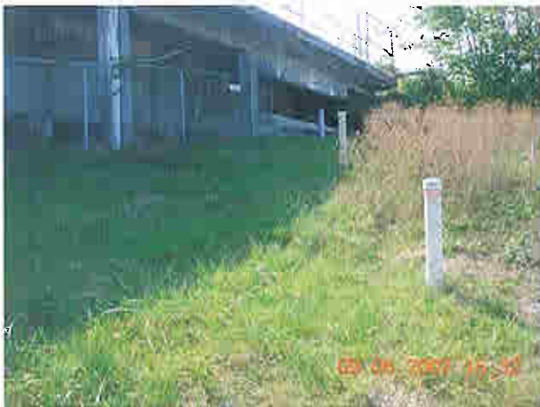
Downstream left embankment and access deck
