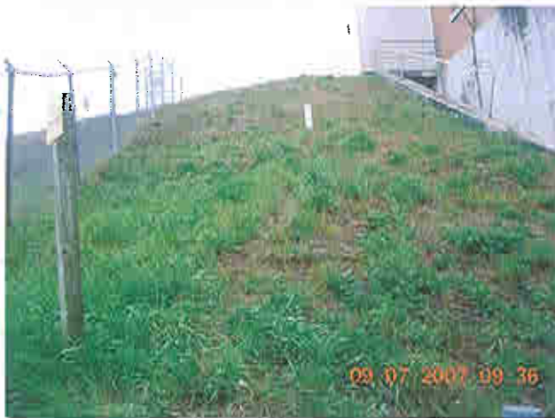
Downstream right embankment slope
