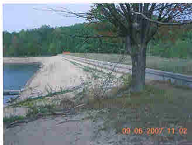
Upstream of detached embankment, note concrete wall
