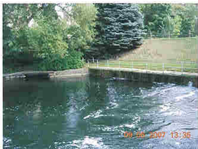
Downstream side of principal spillway
