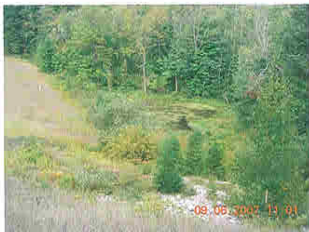
Downstream of detached embankment, note stone
