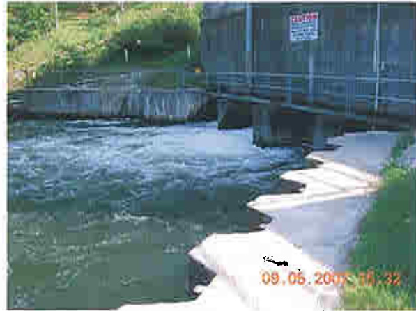
Downstream side of powerhouse
