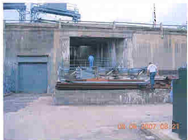
Downstream side of road
