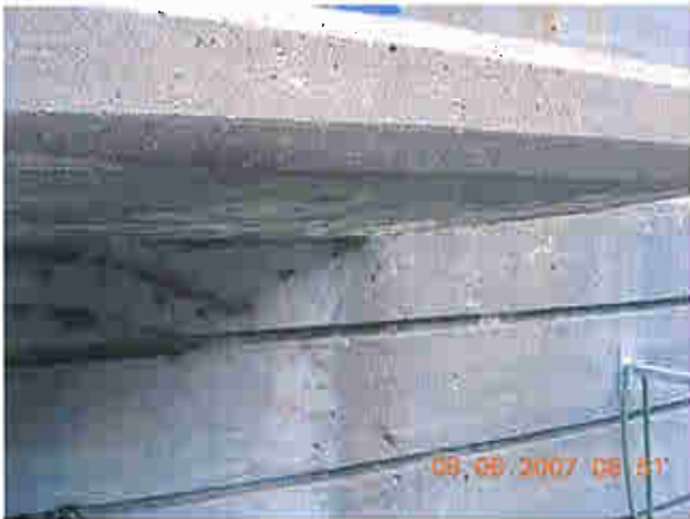
Under deck at entrance to powerhouse, appearance of recent concrete repairs
