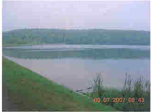
Upstream slope and impoundment at left embankment
