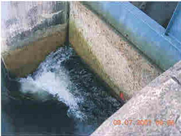
Downstream of log chute spillway
