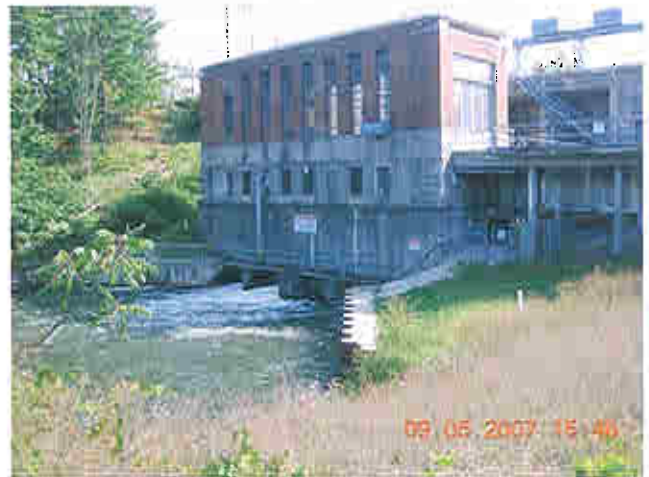
Downstream side of powerhouse
