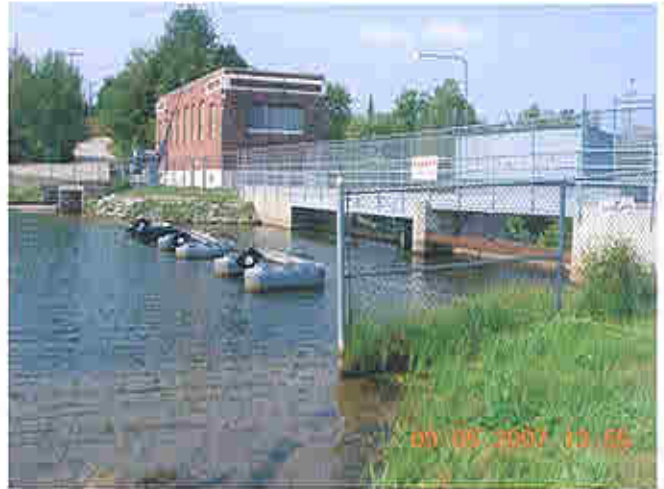
Upstream side of dam, view from right embankment
