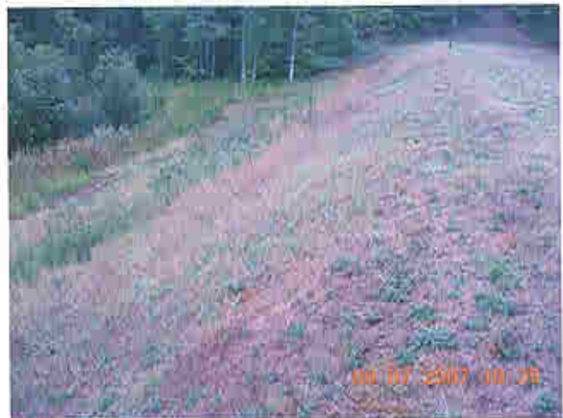
Downstream slope of right embankment
