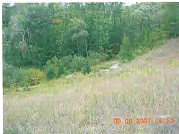
Detached earth embankment downstream slope, right end
