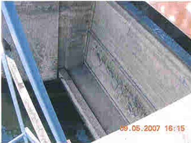
Gate at spillway
