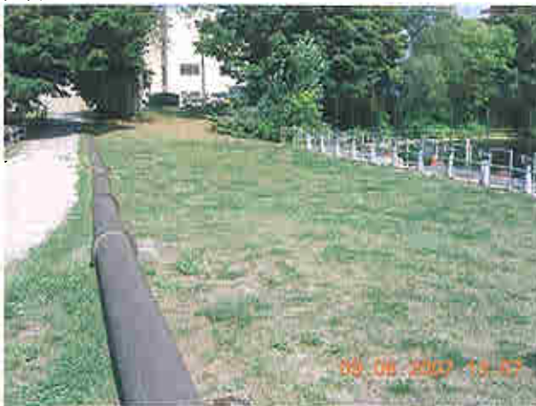
Upstream slope at principal spillway, view looking right
