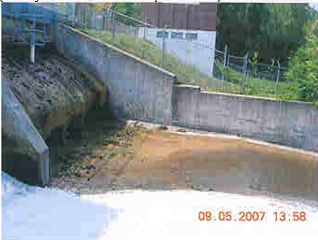
Downstream side of stop log spillway
