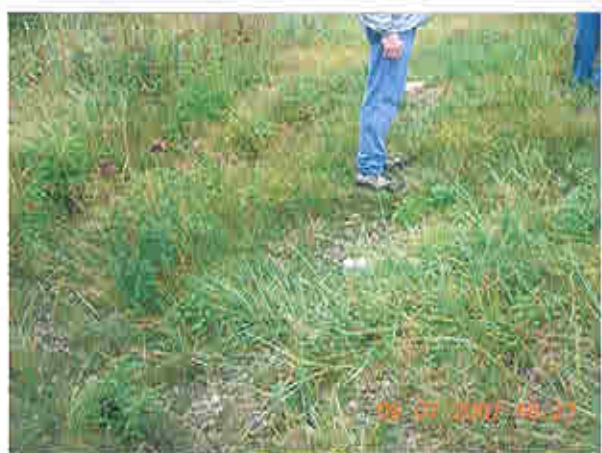
Downstream slope of right embankment
