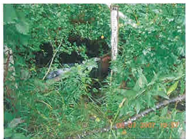
Measurement weir- assumed to measure seepage and natural stream flow
