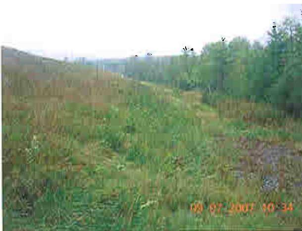
Downstream slope of right embankment
