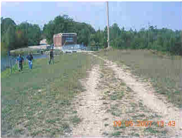
View from right embankment, looking left
