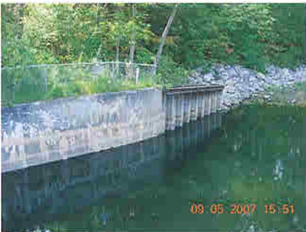
Downstream of spillway, view of left abutment
