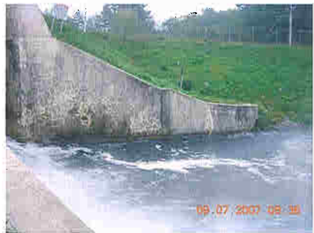
Left downstream abutment and embankment
