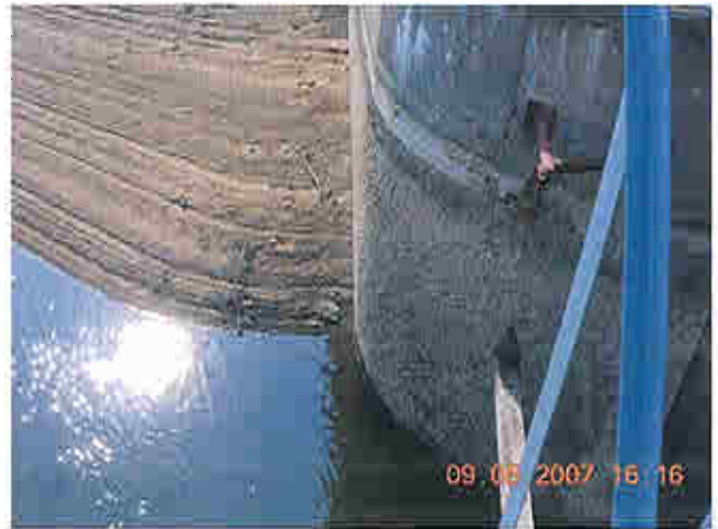
Right upstream abutment
