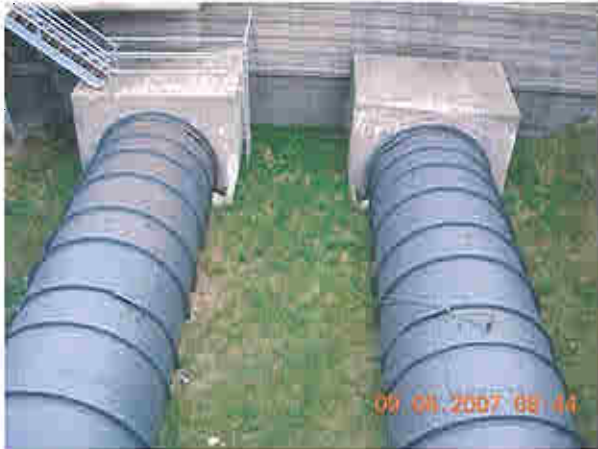
View looking downstream at base of powerhouse and penstocks
