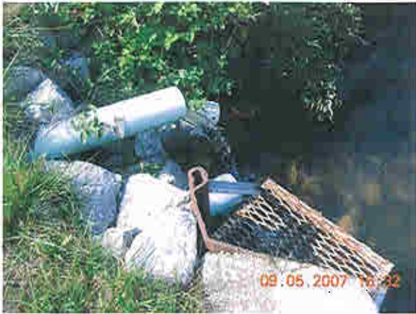
Downstream left of powerhouse, note water flowing
