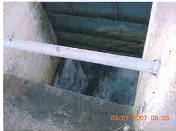
Downstream side of log chute gate
