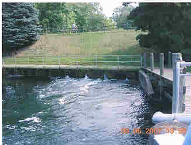
Downstream side of principal spillway
