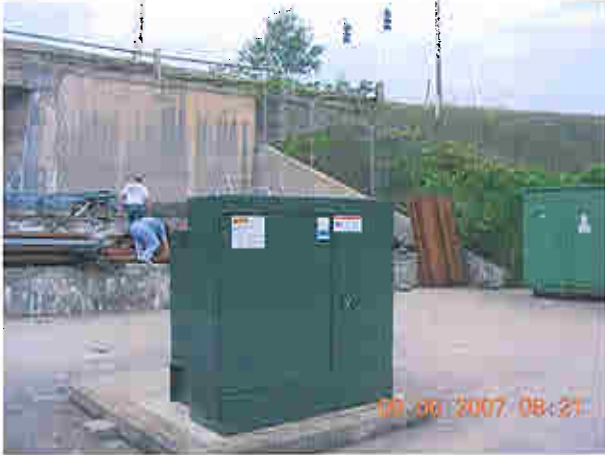
Downstream side of road abutment
