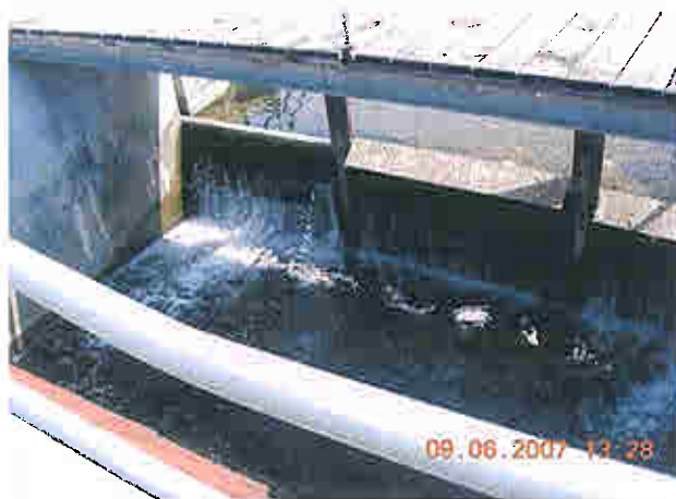
Downstream side of stop log overflow section of auxiliary spillway
