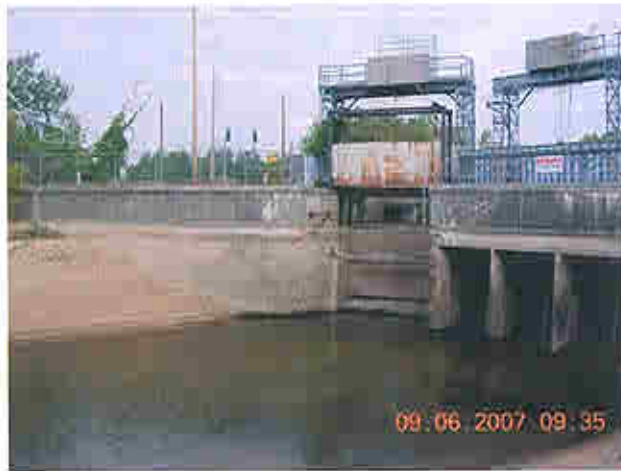
Upstream face of dam
