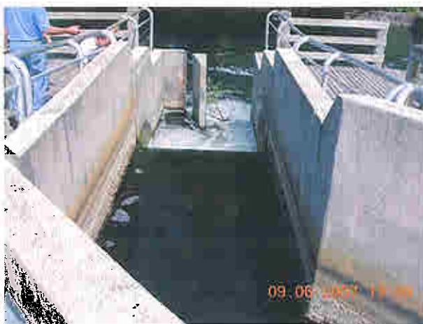
Fish ladder, view looking downstream
