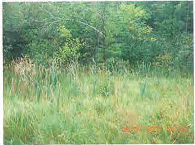
Downstream of downstream slope of right embankment
