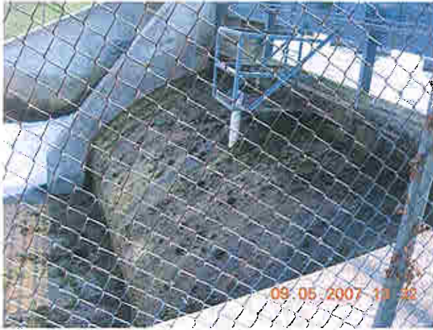
Downstream side of stop log spillway
