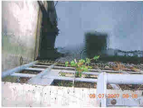
Upstream side of trash racks at tainter gate spillway
