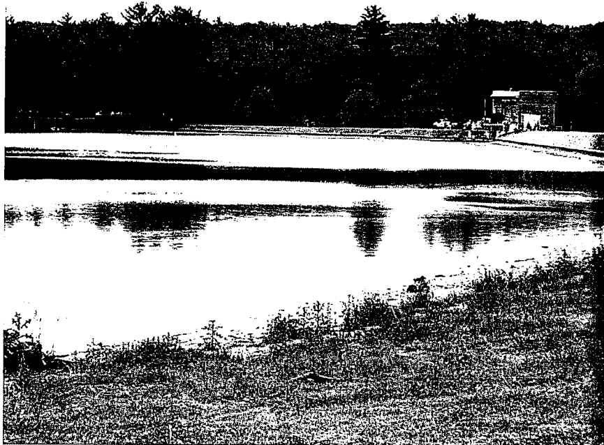
Photo 1 – 6-19-08 - View of left embankment dam and powerhouse/spillway structure from right abutment.
