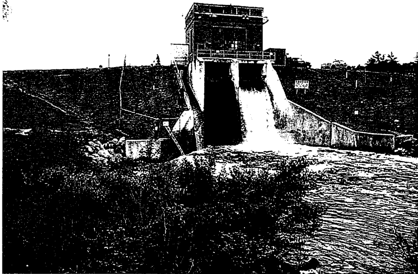
Photo 13 – 6-19-08 – View of downstream side of powerhouse/spillway structure and left and right embankments. Note upper spillway gates and log chute.
