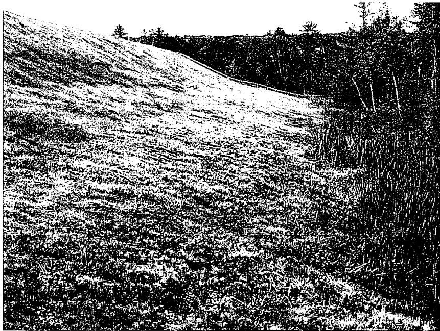
Photo 8 – 6-19-08 – View looking left from toe of right embankment. Note that dark green grass identifies elevation where the phreatic surface is close or at the ground surface.
