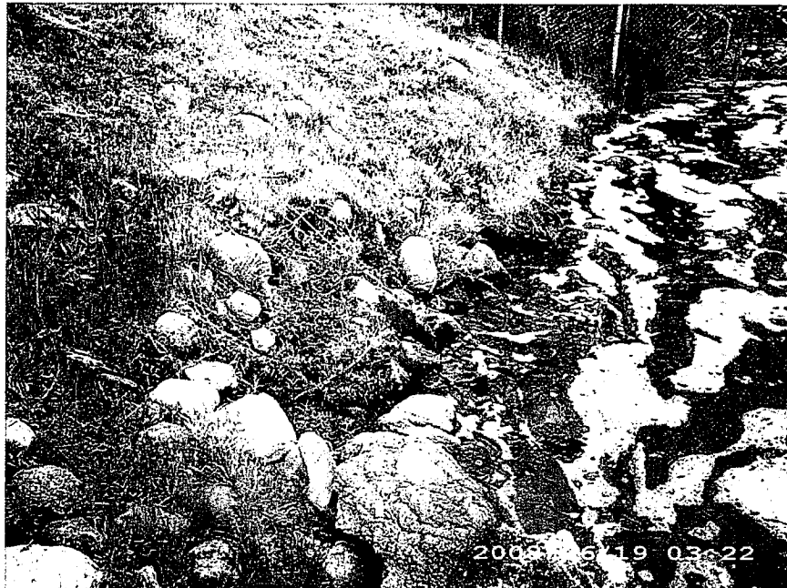
Photo 3 – 6-19-08 – Toe of natural soil to left embankment contact near end of spillway. Note soil erosion at toe of slope. Seepage flow was evident in this area and above.
