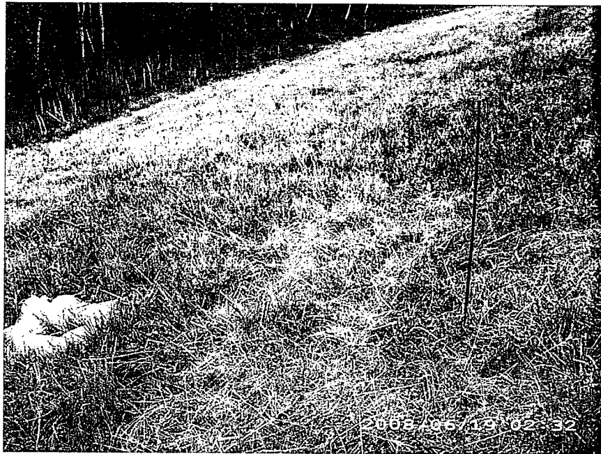
Photo 9 – 6-19-08 – View of rebar probe and area where sand bags were used to confine a former seep. The seep was not flowing but wet.
