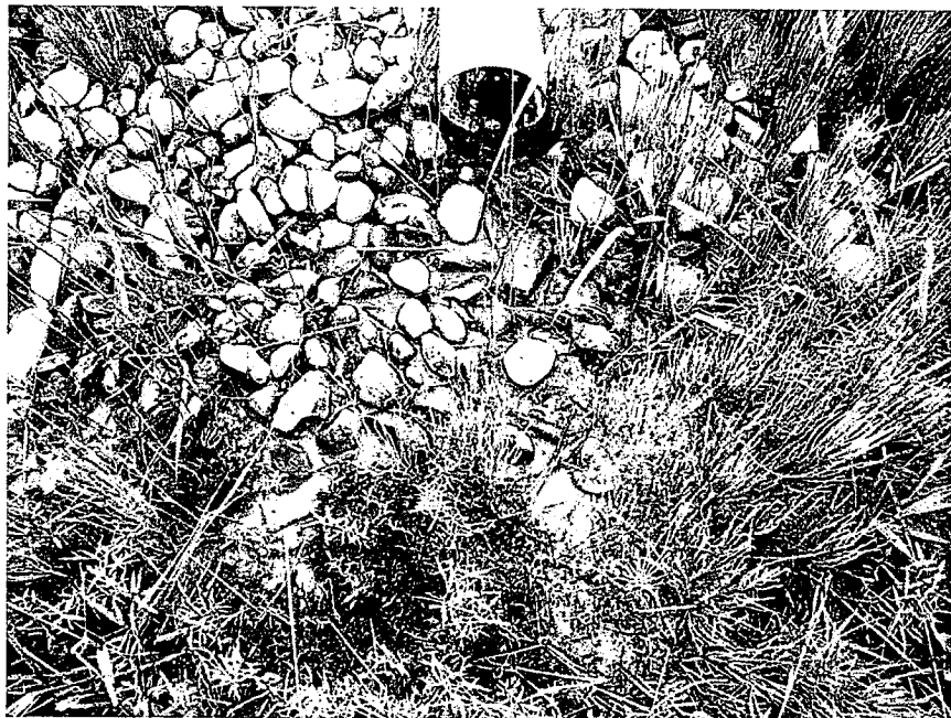
Photo 10 – 6-19-08 – View of typical drain pipe along toe of right embankment. Note sand deposits within grass.
